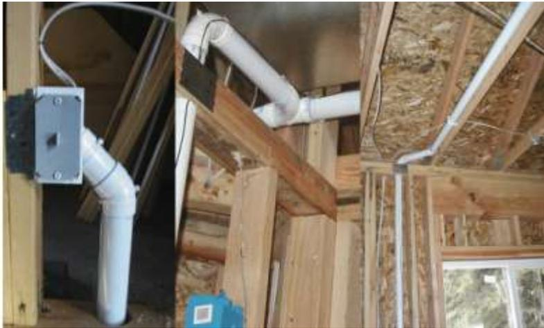
If you are *health conscious* but can't afford a full system initially, 'plan for the future' by installing the ducting only, at the framing stage of construction.
